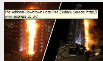
The Address Downtown Hotel Fire (Dubai). Source: http://www.express.co.uk/
